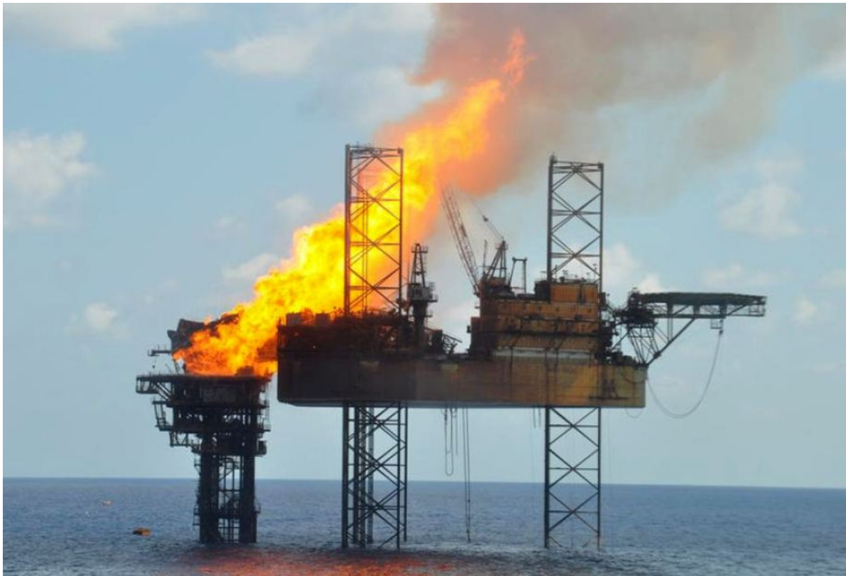
Figure 1. Montara oil platform ruptured in 2009 (Lannin, 2016)
